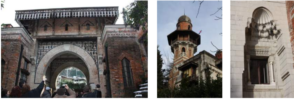
View of the Entrance Building, the Tower-minaret, External Wall Detail (Lombardi, December 2012)
