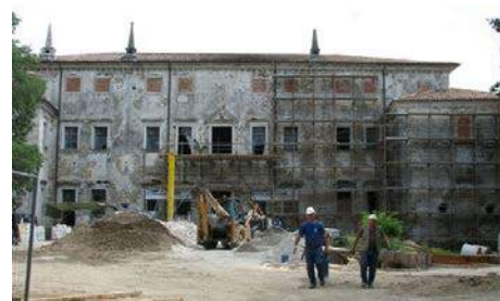
During Renovation (www.skyscrapercity.com)
