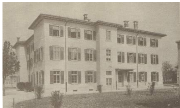
Above: Southern Facade in 1933 (OPP, 1933)
