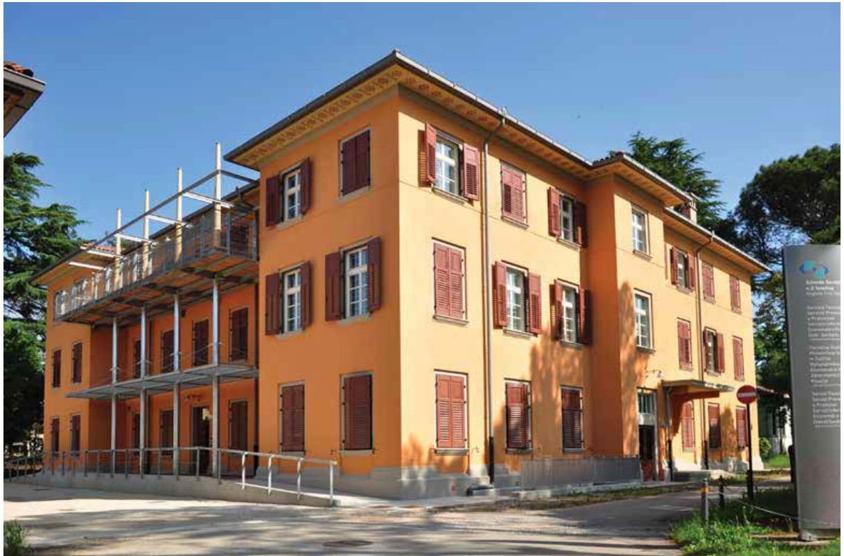
View from the South-west Corner (Starassociati, 2016)
