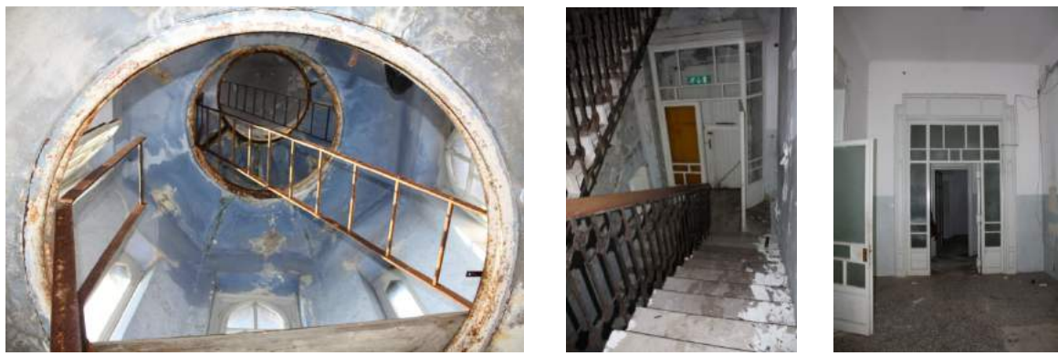
Inside the Tower; the Secondary Staircase; First Floor (Lombardi, September 2012)
